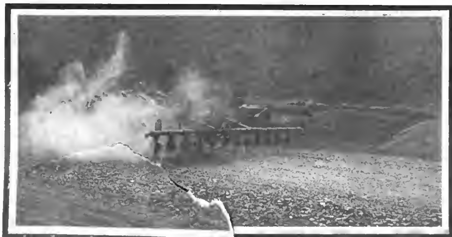
Splendid view of machine used in Massachusetts for spraying hot oil under pressure upon roads
